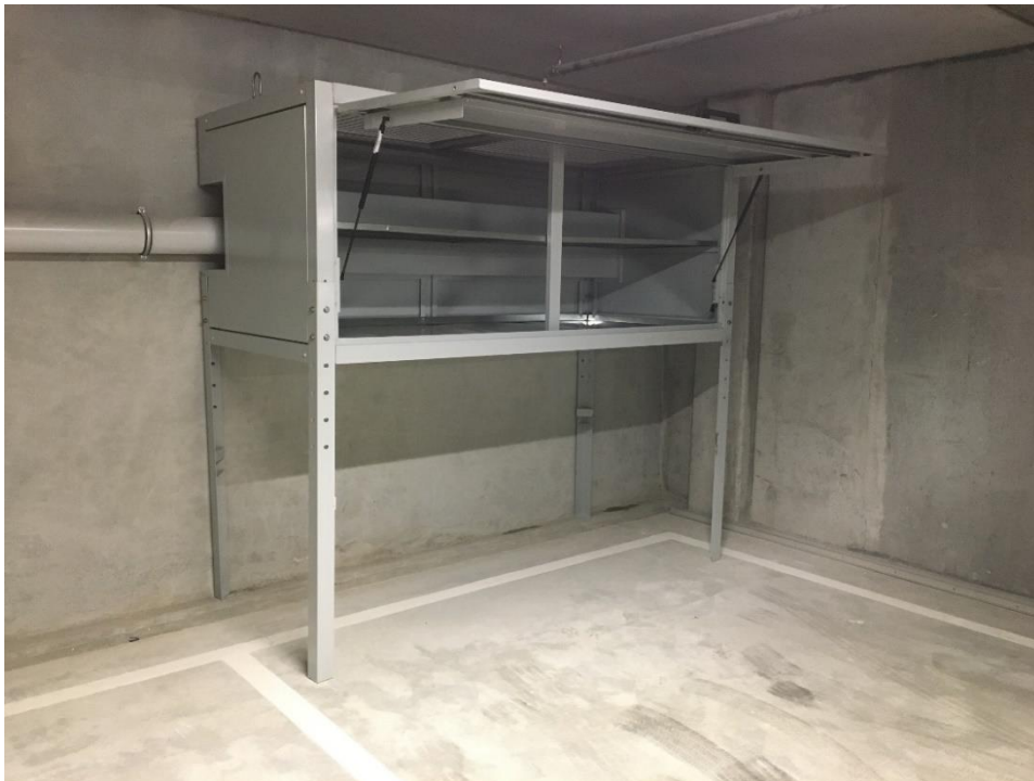
Example of Top Hinged Door Unit with Pipe Clearance Cut Out
